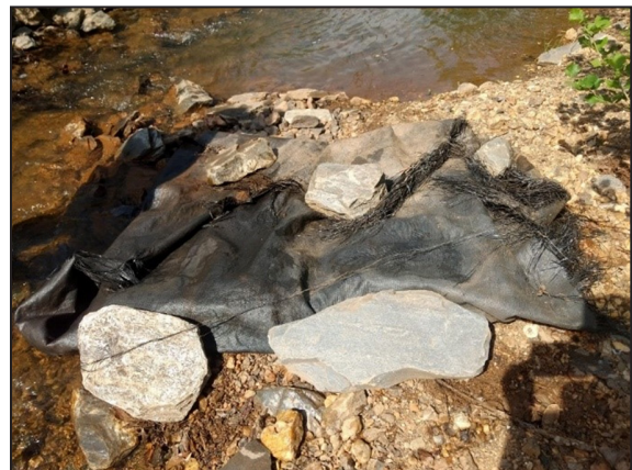
FIGURE 2. Representative snake structure constructed of black landscape fabric folded over with rocks between the folded material as well as on top to hold the structure in place when stream levels rose after storm surges. (Photographed by Rachel Beiler).
