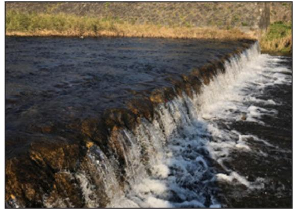
**FIGURE 2.** A weir in the Kamo River, Kyoto, Japan. The structure is made of concrete, has a height of 54.3–84.3 cm, and is used to reduce the effects of flooding. (Photographed by Koshiro Hara).
