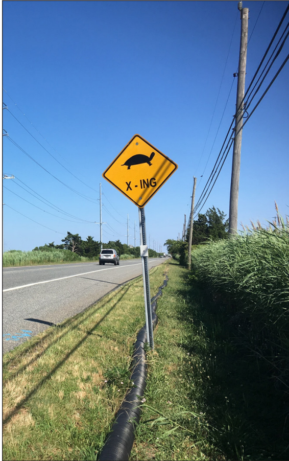
FIGURE 4. Corrugated plastic tubing barriers installed along portions of the road transect in Cape May County, New Jersey, USA. (Photographed by Addie Schlusset).
