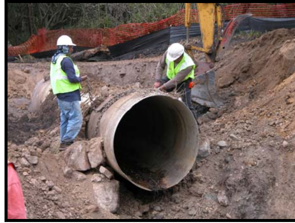
FIGURE 2. Removal of a culvert at Mt. Vision Road, Point Reyes National Seashore, California. We found no Dicamptodon ensatus under this culvert even though the cavern on the underside of the culvert was similar to those at both the Estero and Glenbrook sites. However, the Estero and Glenbrook culverts were much wetter and provided better amphibian habitat. At the time of this photograph, rock and soil had been removed from the top and sides of the culvert, but nothing had been disturbed below the lower lip of the culvert.
