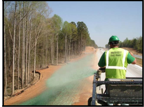
FIGURE 4. Example of a hydraulically applied erosion control product (HECP) being applied in-situ. (Photographed by Marc S. Theisen)
